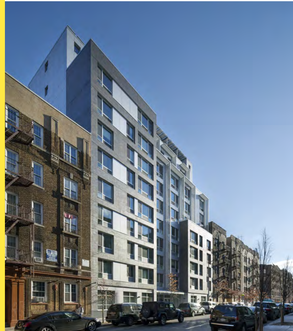
Completed, Creston Ave, Bronx, NY
