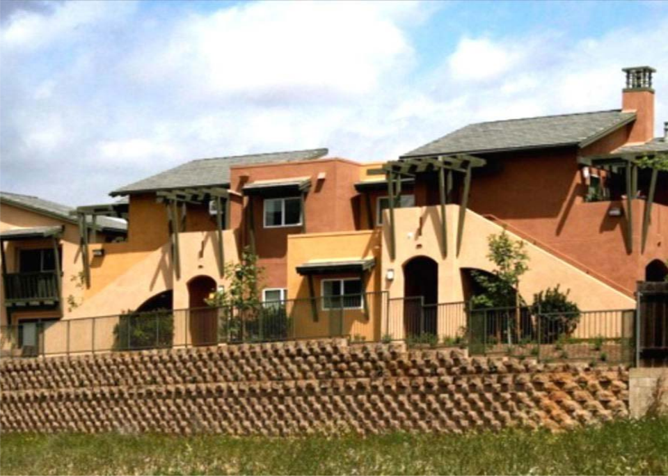
Solara, San Diego Zero Energy Affordable Housing
